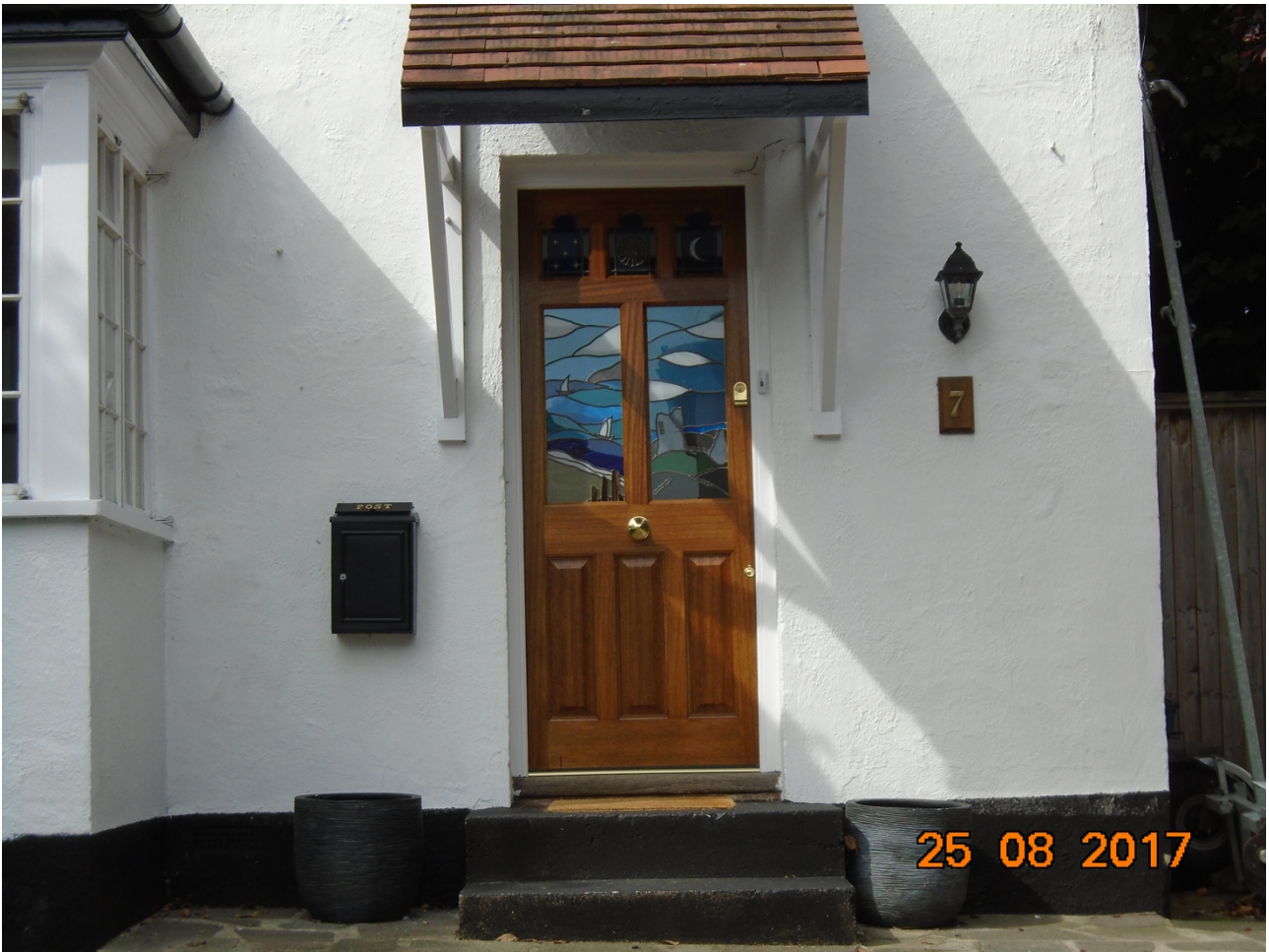
7 Canvey Road - Unauthorised Front Door
